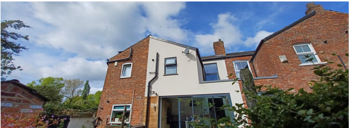
Figure 6. Rear roof of property.
