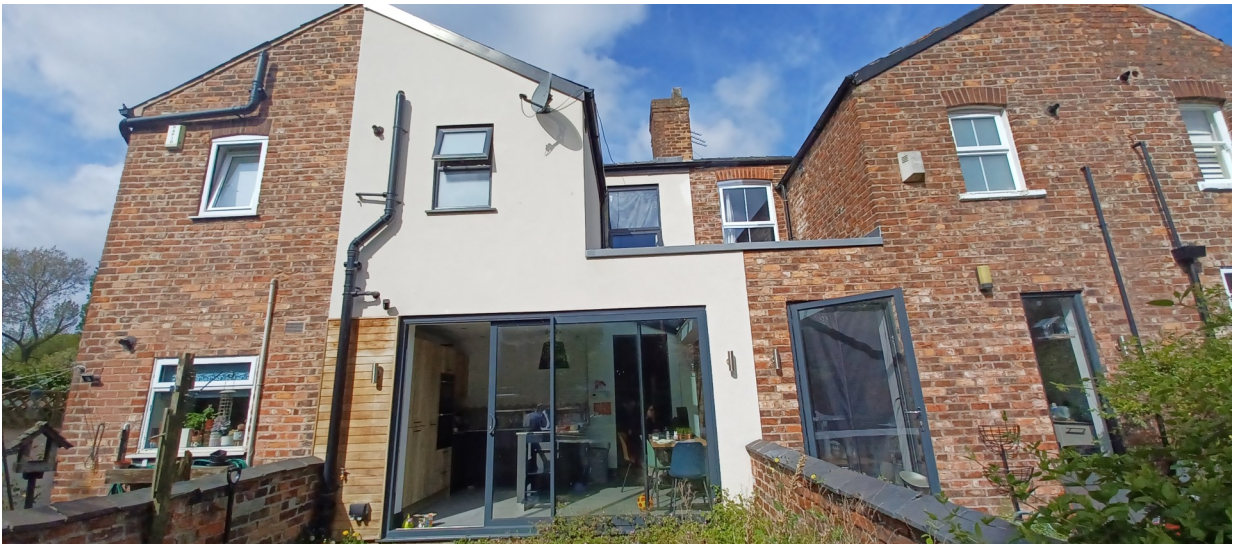
Figure 4. Rear view of property.
